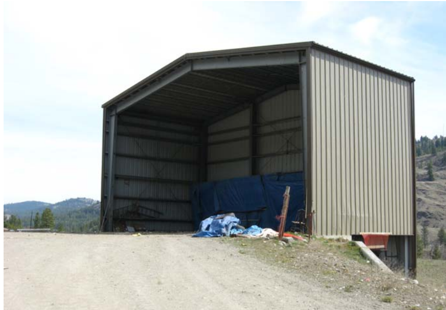
Figure 9.1 Torboy Transfer Station
